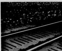
Underdrain system of the International "Wagner Bottom" type. Slotted concrete blocks fit closely in between the distributing laterals.
