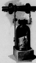
International Pressure Coagulant Feeder with Venturi Proportioner
